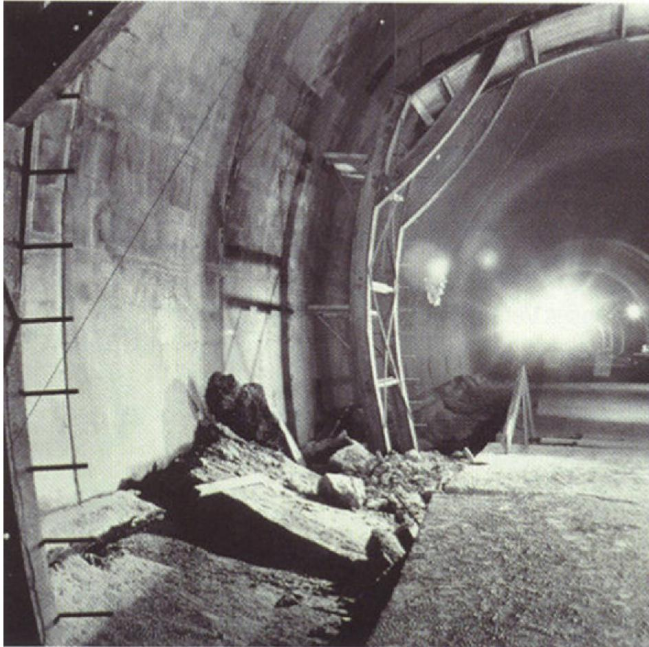
Heave in a tunnel excavated in sulphate bearing rock (Belchen tunnel)
